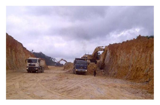
**Emerald Mining Venture:** Mining the ore, haulage and stock the ore, load the washing plant, recover the mined land according to Minerals commission directives.product throughout the area.
